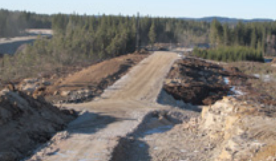
Almost the entire Rural Road has been filled up with rubble in preparation for asphaltting. March, 2013.
